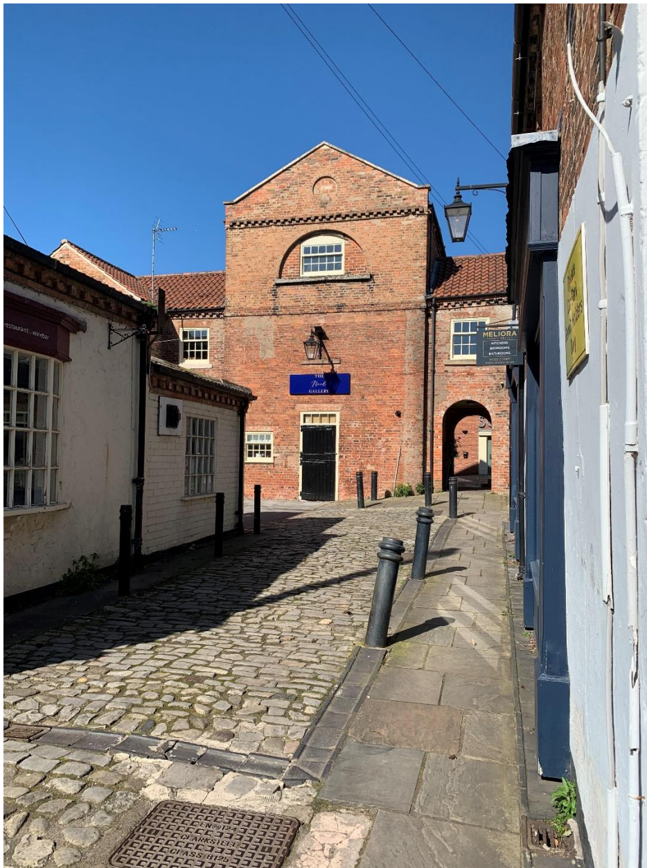
The remaining buildings of the Swan Inn viewed from Swan Street
