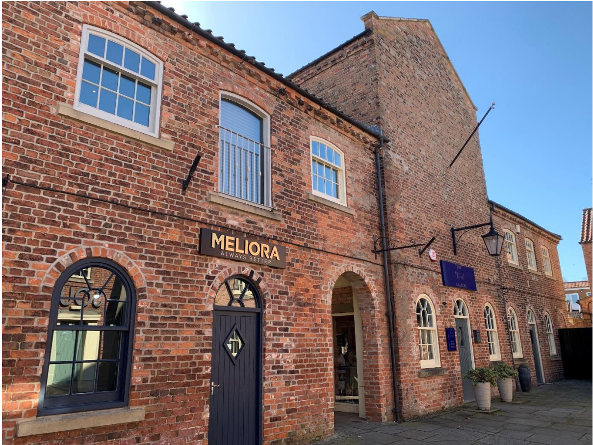
The Courtyard elevation of the dovecote and stables, the only remaining parts of the Swan Inn
