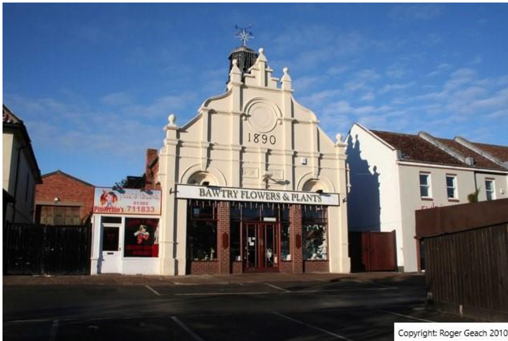
The Old Town Hall, 17 Market Place, High Street
