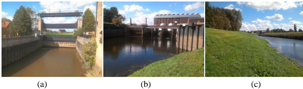
Figure 6; (a) The 2016 replacement tidal sluice at West Stockwith; (b) The Idle pumping station, sluice gate to the left; (c) The enormous pound lock created between the two barriers. Images 2016 © M. Newman, reproduced with permission.
