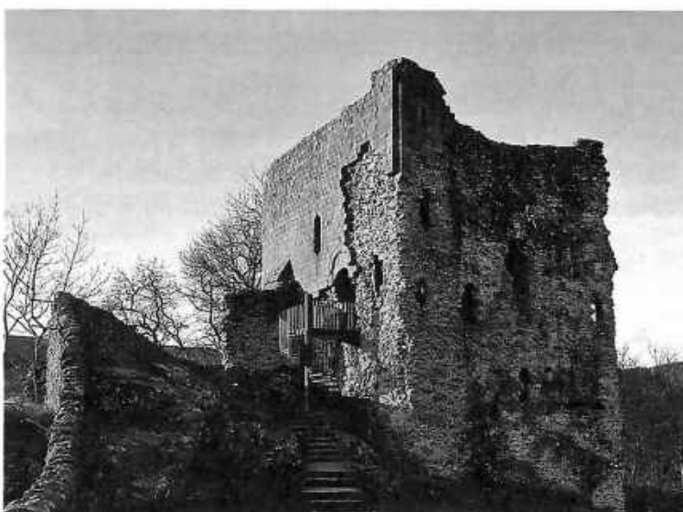
Pevelevil Castle, left, formerly known as High Peak Castle, now in ruins on a ridge above Castleton. The castle was granted to John of Gaunt with other properties in exchange for Richmond Castle in 1372. John of Gaunt had little use for High Peak and had some material, such as lead, removed and taken to Pontefract Castle in 1374. However, the keep, built by Henry II, was retained to serve as a court house.
