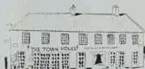
8. The Town House Built in 1691 for the Dawson family who were merchants trading as far afield as the Baltic. Prior to its present use it was known as Barton's Garage.
