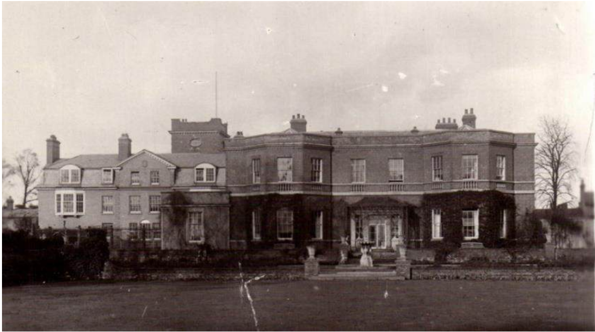
Fig 11 - The south elevation of Bawtry Hall prior to RAF use
