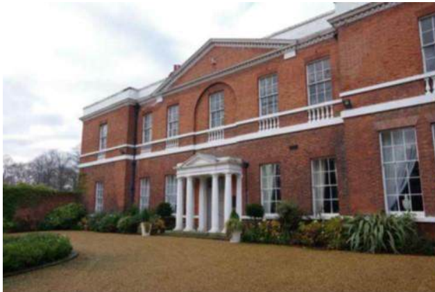
Fig 2 - A recent image of Bawtry Hall - front (east) elevation
