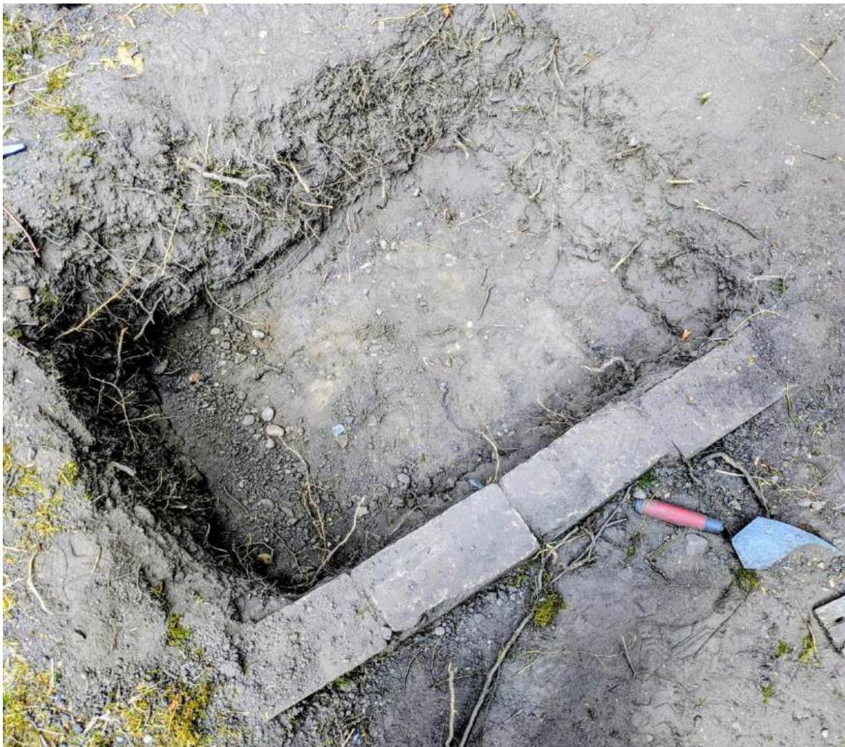
Photograph 4 Trench area two.
